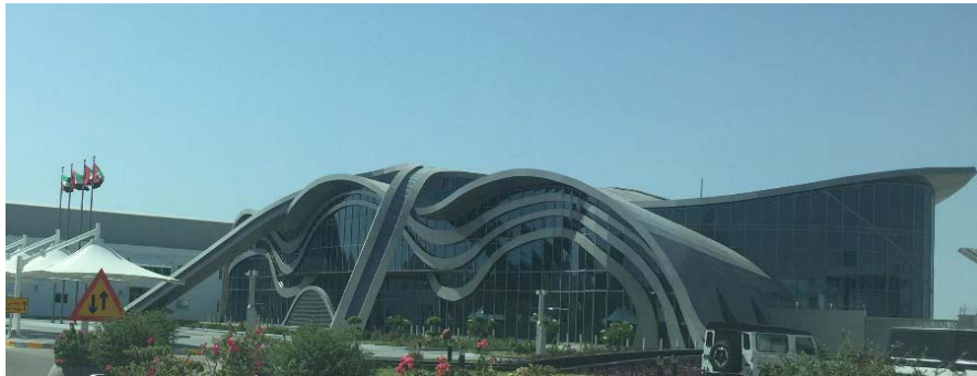
Landside view/PV panels on the roof
