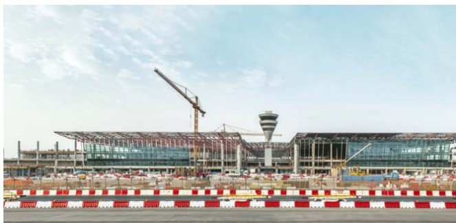
New Passenger Terminal Building Construction Site.
