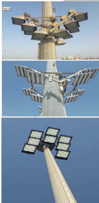
New LED type R4 Vs HPS Light systems and New LED lights Type F32
