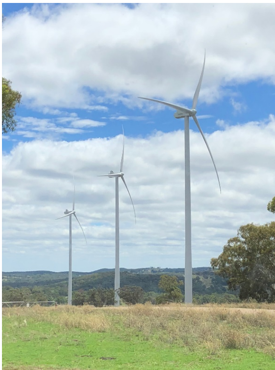
Three operational Sapphire turbines
