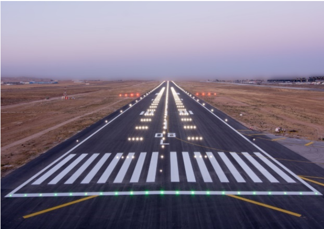
Approach light-08L-North runway
