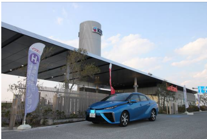
FCV and Hydrogen station
