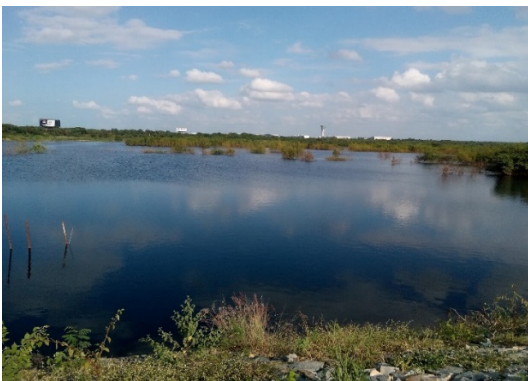
Rainwater harvesting structure (R2) at the Airport
