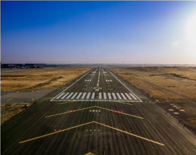
North runway –day light view
