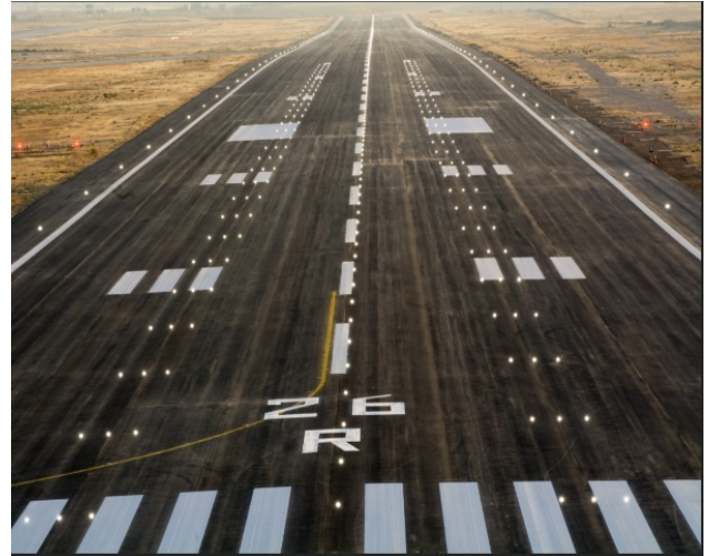
Approach light-26R-North runway
