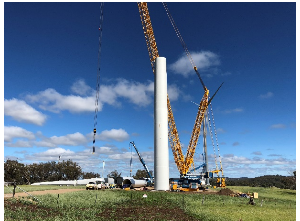
A Sapphire wind turbine being erected
