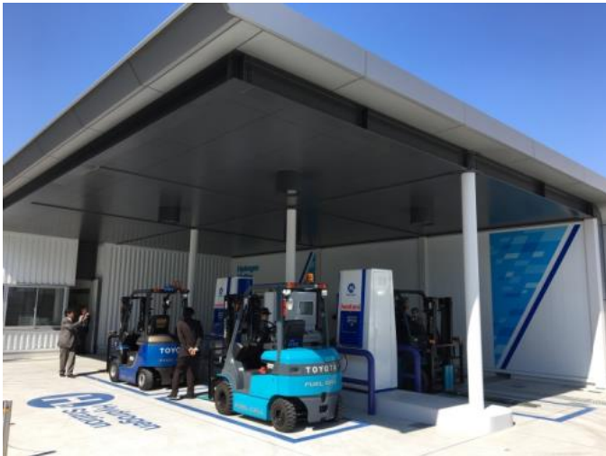
Hydrogen station for industrial vehicles
