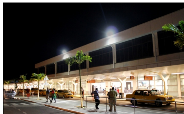
Replacement of all lightings with LED lights and is managed through the BMS.
