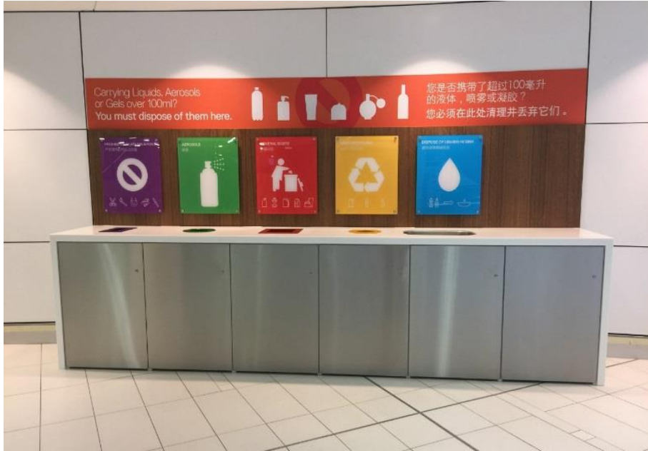
Image of final installed waste station
