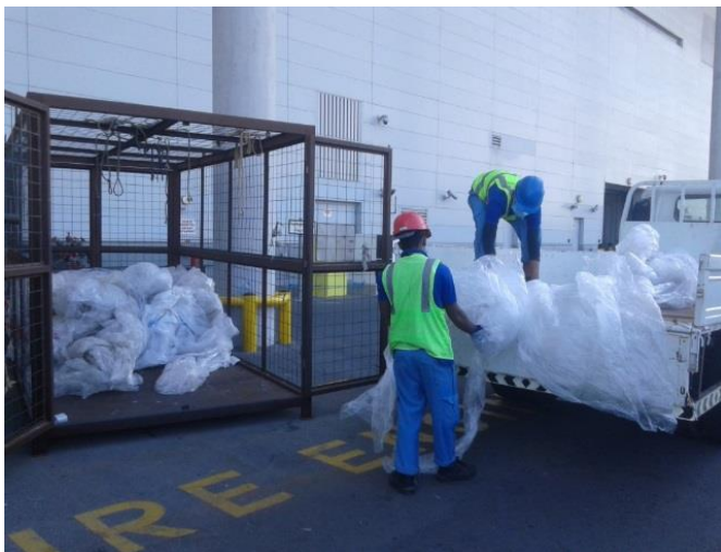
Two staff in the process of transferring plastic waste from the previous cage and loading into a truck. The plastic waste can easily be blown away by wind creating FODs.
