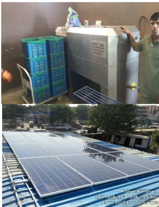
Roof top Solar plant installation(5Kwp) at OWC
