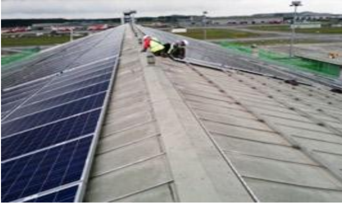
Caption 1 Installation Works
