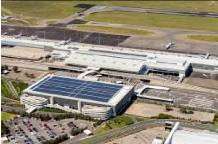
Caption 1 Adelaide Airport 1.17MW Solar Installation
