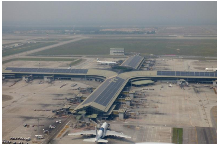
Caption 3 Roof Top, Satellite Building KLIA (4MW)
