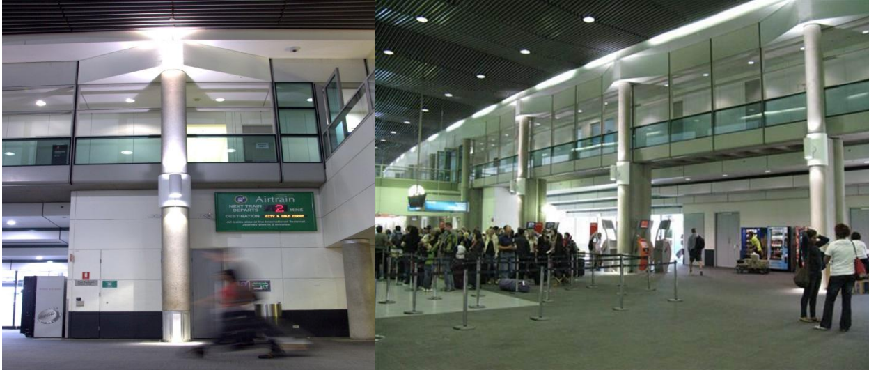
Caption 1 Domestic Terminal Lighting Upgrade Photo
