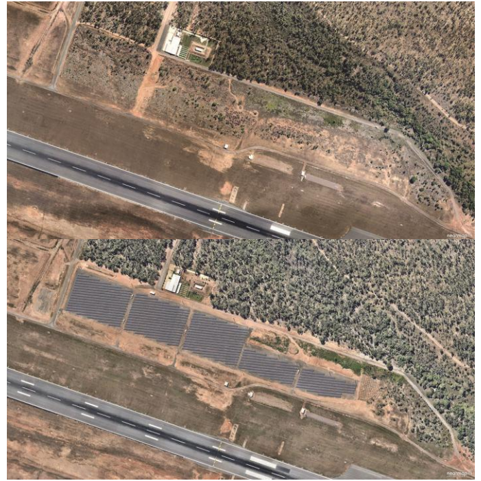
Caption 2 Darwin Airport Solar Project Stage 1, before and after
